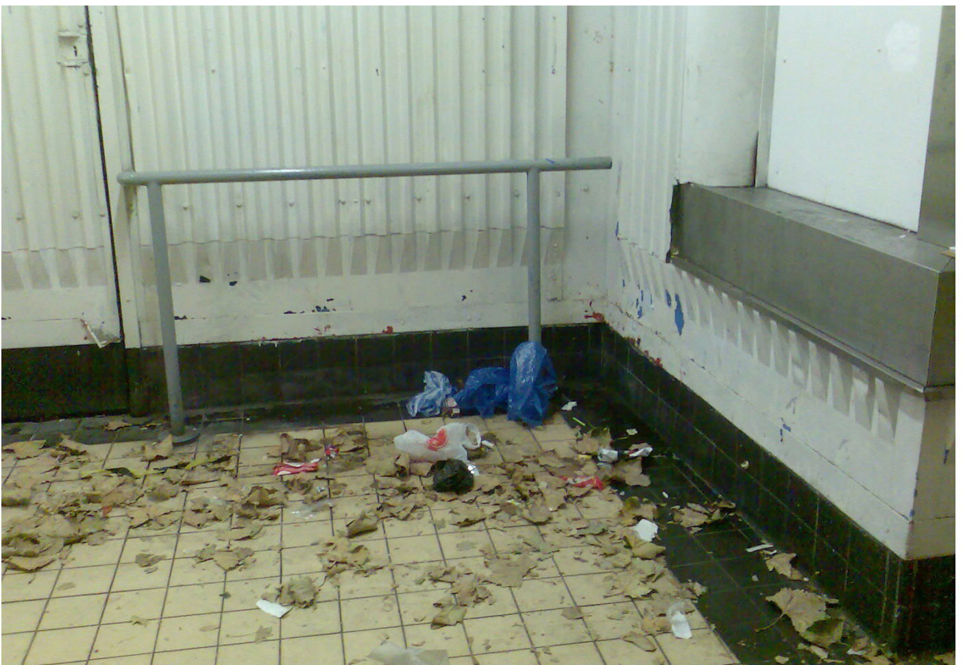
CAMBRIDGE HEATH: The litter-strewn entrance hall in 2007 with the boarded-up and abandoned ticket office on the right. The smell of urine was often so strong people had to hold their noses
